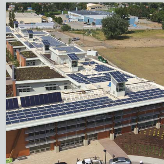
Okanagan College. Photo: SkyFire Energy Inc.
