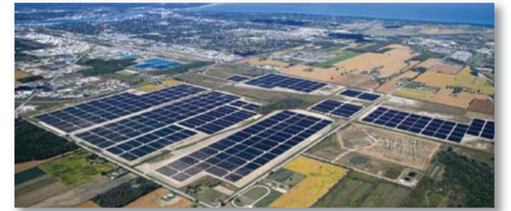
Aerial view of Enbridge Sarnia photovoltaic installation. Photo: First Solar.
